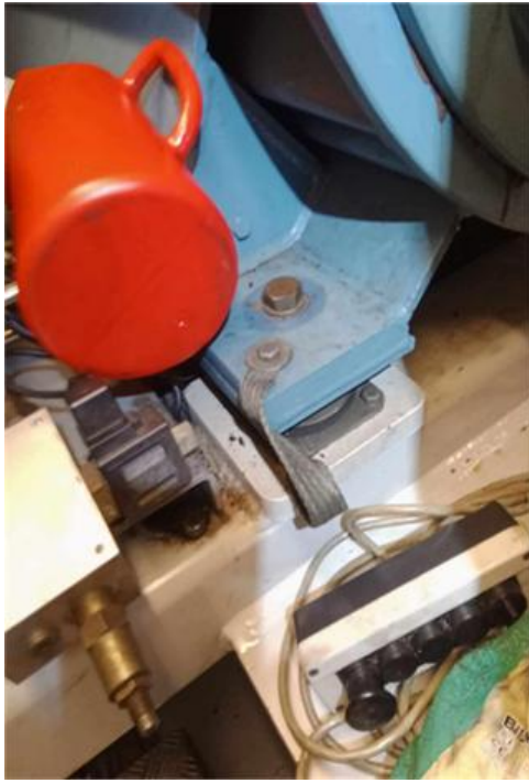
Figure 5: Low-impedance connection between generator mount and tower superstructure ensures that the wind turbine tower tube is fully utilized as a part of the grounding system for the wind turbine.
