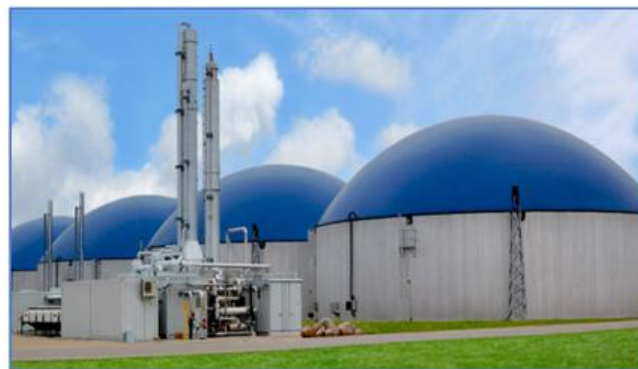
Figure 3: Advance Plant Generating CBG located in Karnataka
