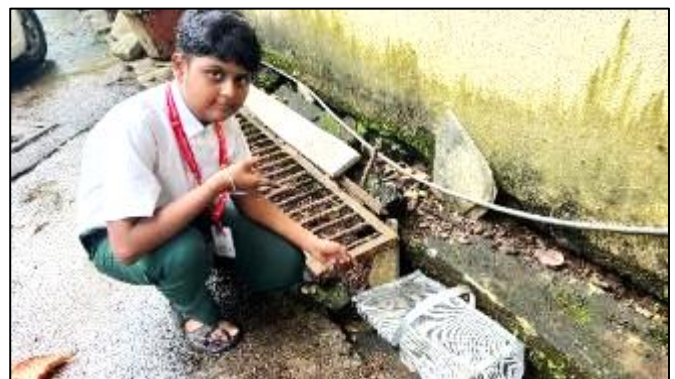
Figure 3: Sewage Cage System placed in an open nala trapping floating waste.]
