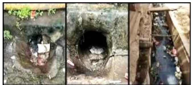
Figure 1: Open kerb scupper inlets along the footpath and open rural nala
