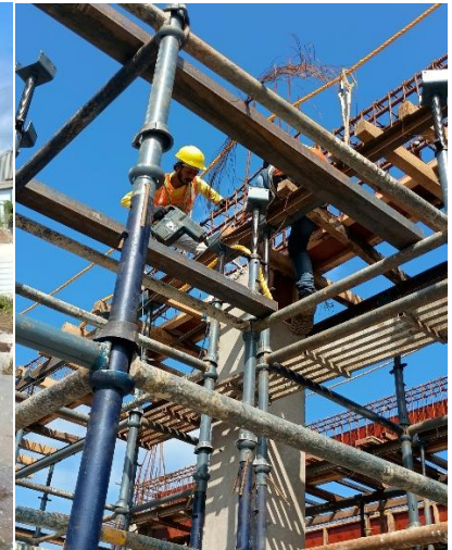
Demolition of Extended Part
