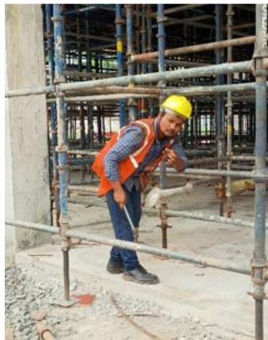
Removing ledger for another work
