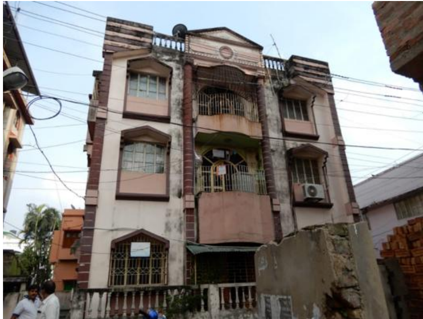
Figure 1: 3-story building where gunshot penetration was reported in the window of the 2nd floor.
