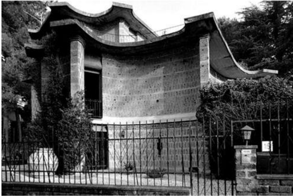
Figure 1: The View of the Baldi house, Rome, 1960. [24].
