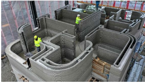
Figure 3: 3D - printed house under construction
