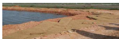
Laying along curved alignment
