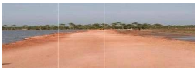
Figure 2: Photograph of partially filled bund
