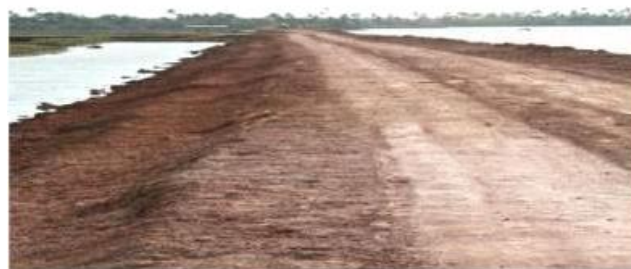
Prepared bed before laying Geotextile
