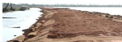
Roll of Geotextile to be wrap around
