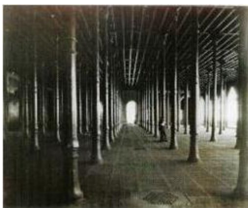
Figure 2: Cast iron structure, interior of González Ortega Market, 1887. Source: CFFSL, p. 191
