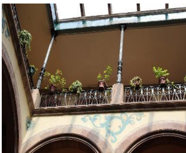
Figure 7: Cast iron columns around the patio, at the upper level. Photographer: IRGO, city of Zacatecas, May 10, 2016
