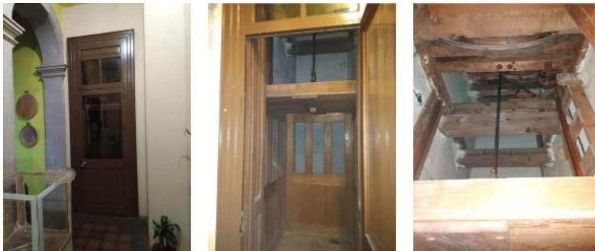
Figure 30, 31, 32: Elevator placed at Benjamín Gómez Gordo's house. This house was evidently remodeled by George E.
