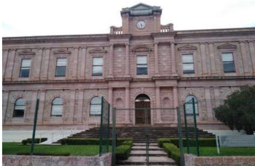
Figure 11: Main façade of the hospital designed by the architect José Noriega. Photographer: IRGO, city of Zacatecas, July 20, 2019.
