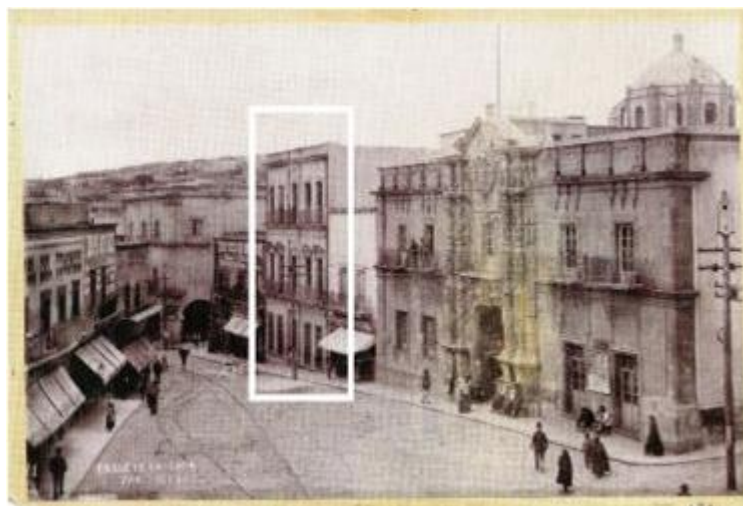
Figure 4: García's house in 1892. The building was refurbished in 1886 using cast iron columns around the patio. Source: CFFSL, p. 247.
