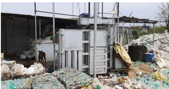
Figure 3: Waste plastic pressing unit
