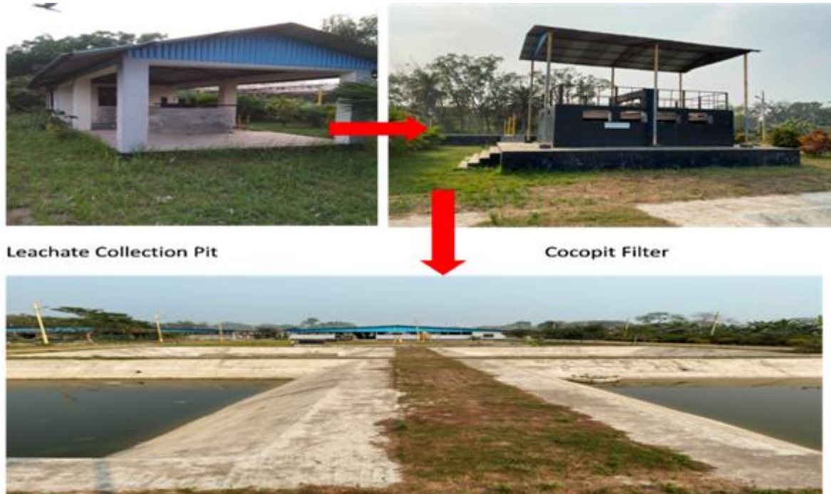
Figure15: Leachate Treatment Plant
