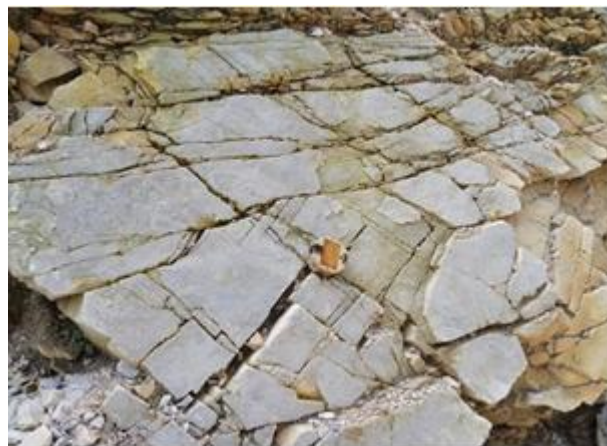
Figure 4: The joints in Sirban Limestone near the landslide having variable Orientation
