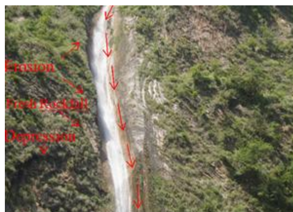
Figure 11: Deflection in the waterfall and presence of depressions in the waterfall area
