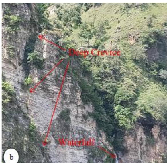
Figure 10 (b): Enlarge view of the Crevice developed at site shown in figure 10-a.
