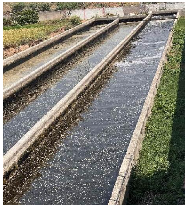
Figure 3.6 --- Chlorine channel Process
