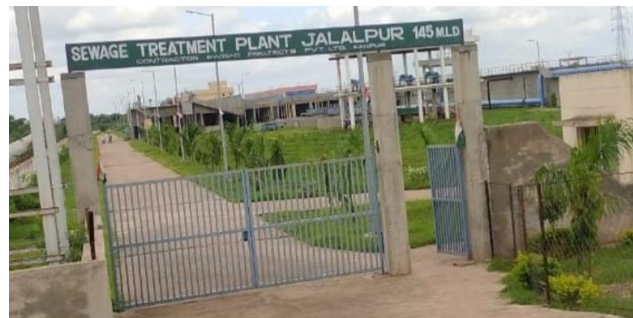
Pic 1: Entrance of STP plant
