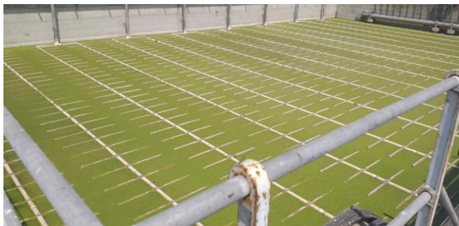
Figure 3.4: Aeration from Bottom
