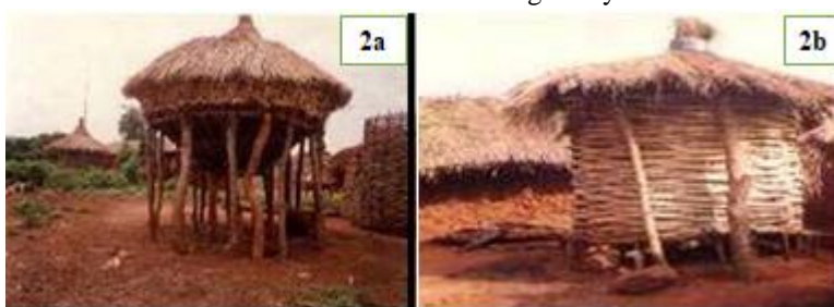
Figure 2: Storage structure in Togo (Akpavi andal., 2007): 2a "Ava" type granary at home; 2b Huidza type granary made with bamboo slats ( Bambusa vulgaris ).
