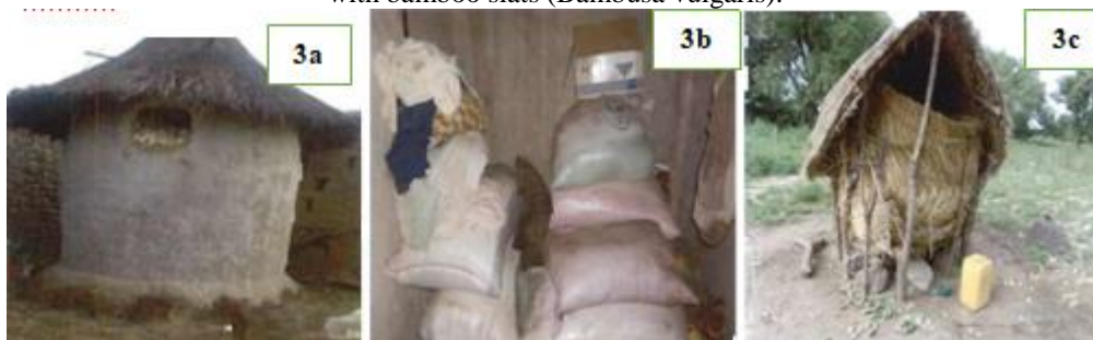
Figure 3: Example of maize storage structures in Burkina Faso (Somda, 2016): 3a: Banco granary; 3b: Bagged storage in a dwelling house; 3c: Straw granary
