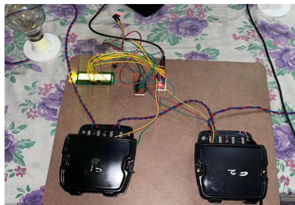
Figure 3: Prototype of Implemented Smart Energy Meter
