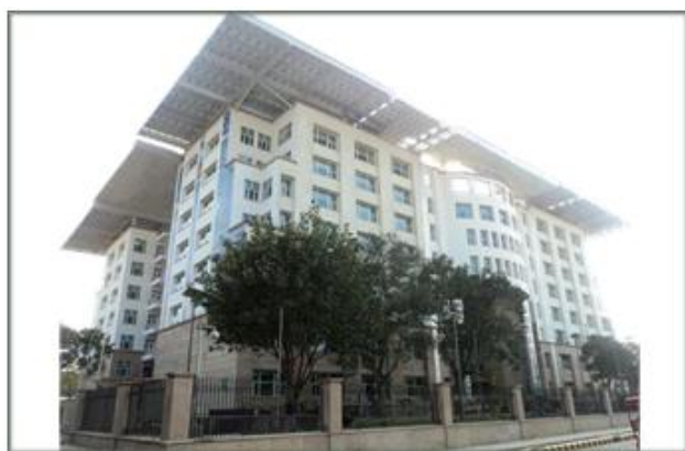
Figure 3.1: Indira Paryavarn Bhawan (source: https://nzeb.in/wp-content/uploads/2015/10/Intro_IPB.jpg )
