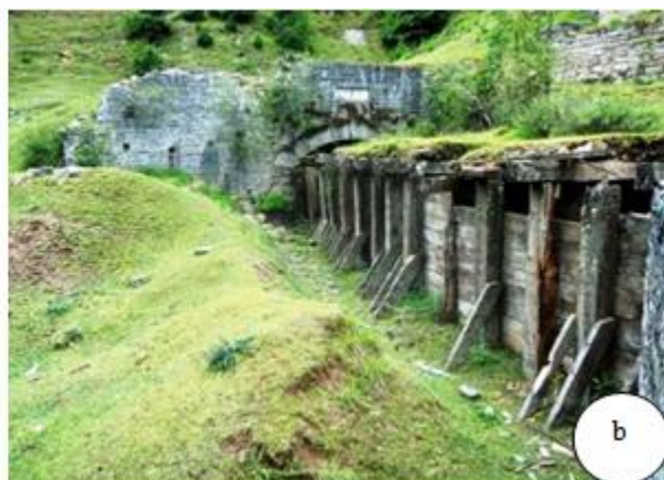
Figure 10: (a) Mohra Hydel Project Distt. Baramulla (b) Wooden Flume, an Artificial Channel (Google images)
