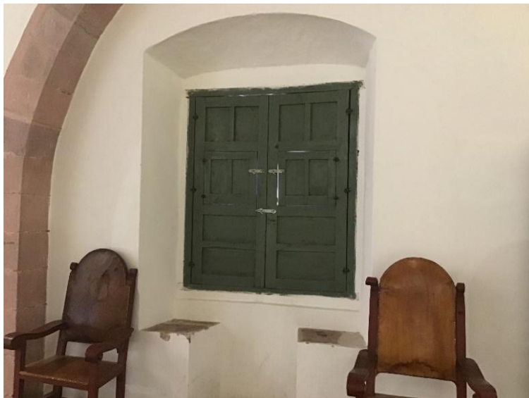
Figure 13: Window with fully closed postigos
