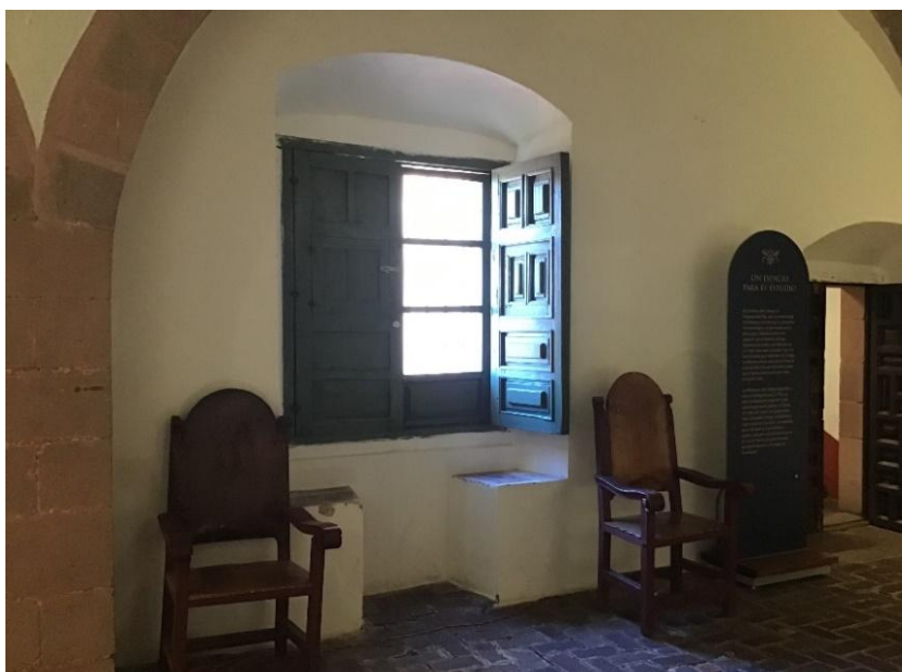
Figure 11: Window with one of the doors that make up the postigo, closed.
