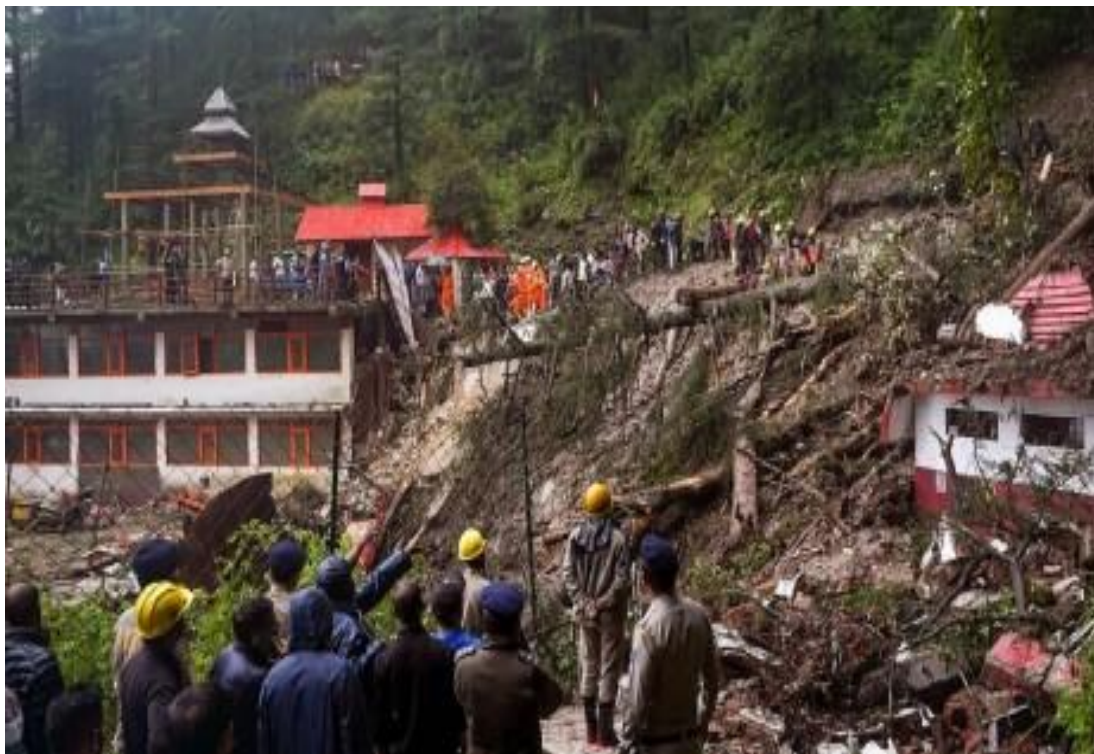
Rock slide occurred along the Shiv Mandir in Summer Hill Shimla
