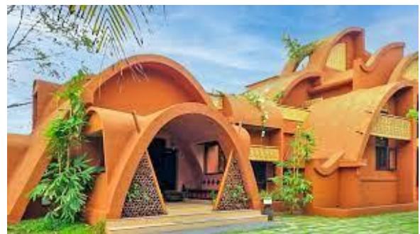
Figure 1: Building built with naturally obtained materials and using sustainable architecture techniques
