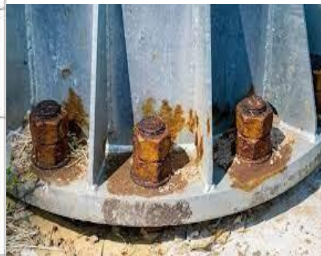
Figure 3: Crevice corrosion between flanges, and bolts.
