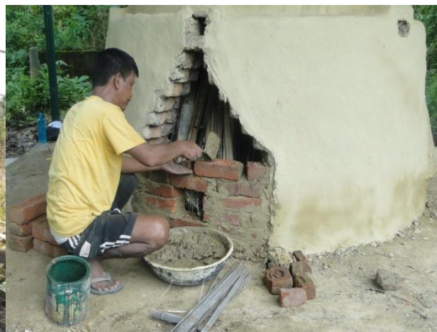
Closing of Brick kiln
