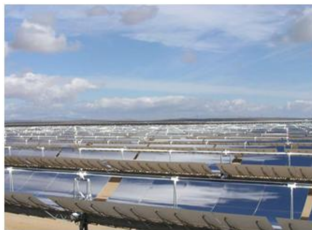
Figure 1: Parabolic troughs collectors of the SEGS plant [3]
