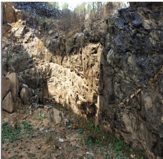
(B) Folded strata exposed beneath new bridge
