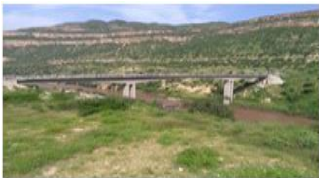
Figure 5: A photo of Abbay Bridge
