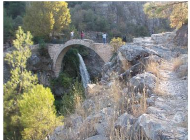
Figure 4: Clanrasaqueduct bridge and remains of rock-cut canal
