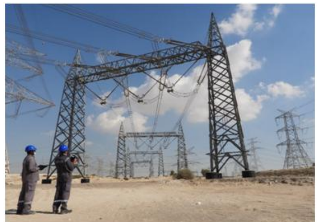
Figure 1: Example of Infrared site inspection using infrared handheld camera
