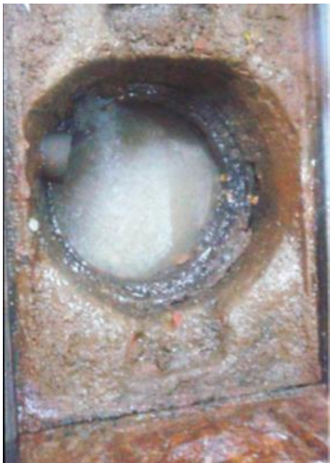
Figure 1: Trial Location 1 - Manhole 1 before application of Biological Solution
