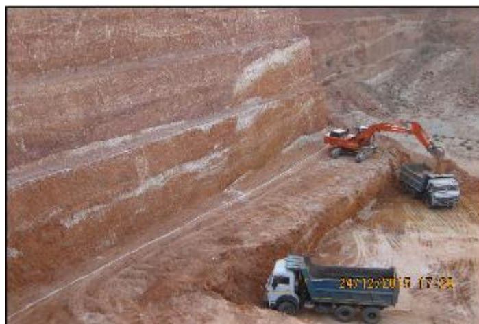
Figure 3: Field photograph showing development of a quarry in Indawara area
