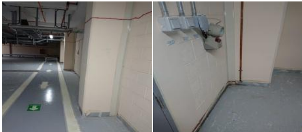
Figure 2: Basement expansion joint area
