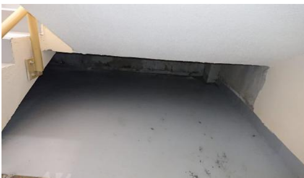
Figure 3: Basement staircase area
