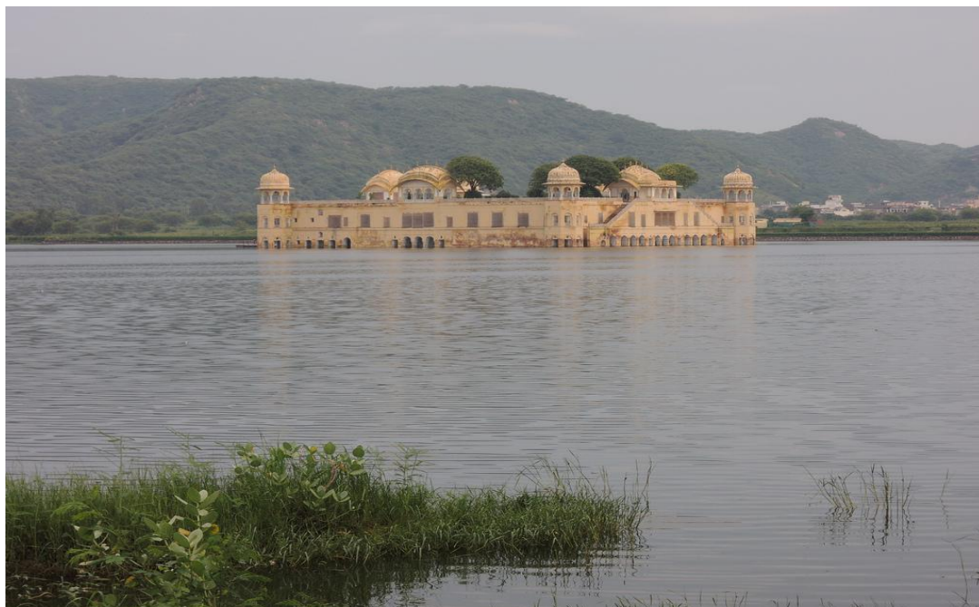
Figure 2: Heritage View of the JalMahal Water Body
