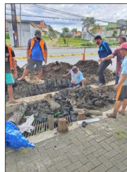
Figure 6: Split DMA Excavation Work
