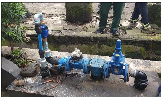
Figure 2: Serial Installation of New Water Meters at Lavalette Hospital
