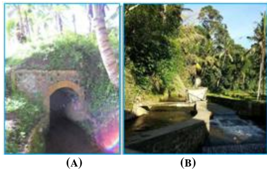
Picture 3.2: Picture A. picture of an irrigation channel in Subak Pulagan in the form of a shadow or tunnel. Picture B. building for water or the so - called tembuk aya (primary canal) that divides irrigation water to the big telabah of Subak Pulagan
