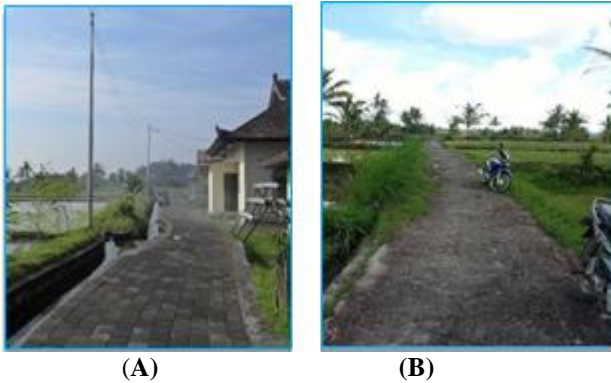
Picture 3.7: Picture A. Photo of a farm road around Bale Subak, where the northern part of the pavement is paving. Picture B. photo of the middle to south part of the farm road with concrete pavement
