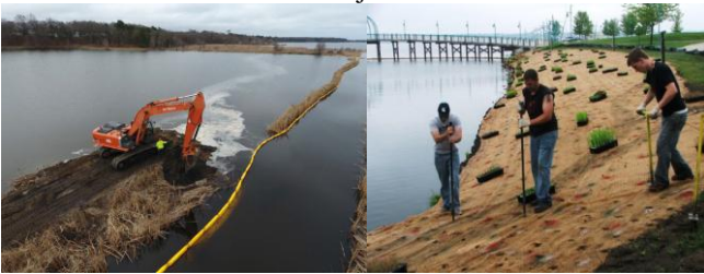
Figure 12: Berm removal Figure 13: Slope stabilization
