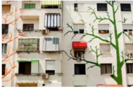
Figure 2: The same building after the intervention
