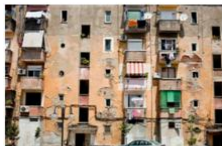
Figure 1: A building in Tirana before the intervention
