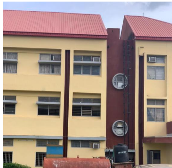
Plate 4: Use of vertical and horizontal fins on the building exterior as a shading device to improve cooling within the faculty building (Source: Authors field work)
