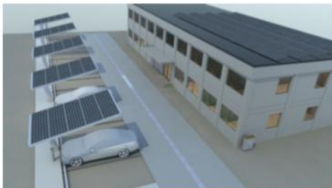
Figure 5.1: Photovoltaic panels powered EVs charging stations where it installed at rooftop and parking lots.
