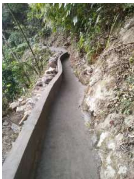
Photo 2 Final work of Single Sided RCC Lining in the canal
