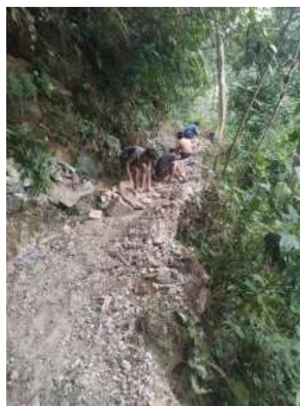
Photo 1 Initial soling on canal by Lepcha Water users
