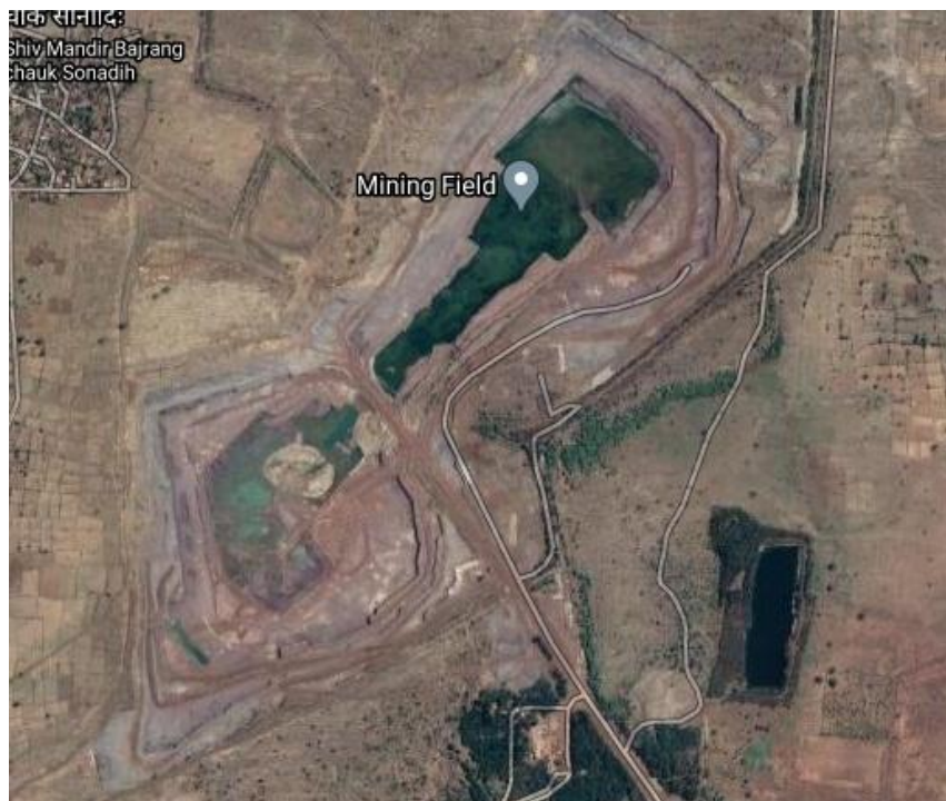
Figure 14: New Karstic feature [Sink hole] in mining area as on 20 March 2020, as per Google
