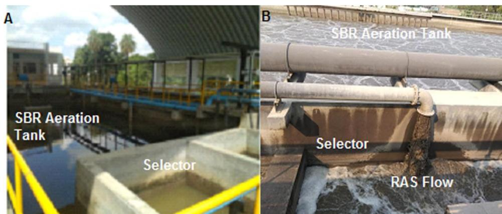
**Figure 1:** (A) Full-scale 3-MLD SBR plant, Roorkee, and (B) Full-scale 120-MLD SBR plant at Goithaha, Varanasi
