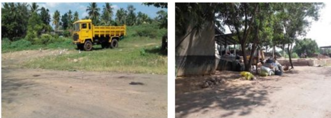
Figure 6: How marshy lands and low-lying lands appear after landfill, Field survey 2016
