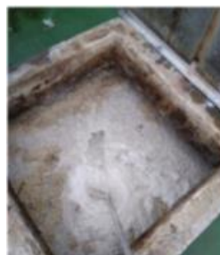
Figure 3: Sludge tank after Bioaugmentation
