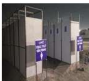
Figure 5: Toilet installed during Kumbh Mela
