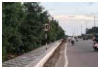
Figure 9: Signboard covered with vegetation
