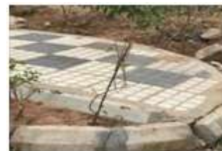
Figure 5: Abrupt closure of Pedestrian track
