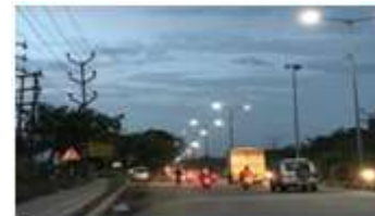
Figure 3: Pedestrian crossing markings are absent on the road
