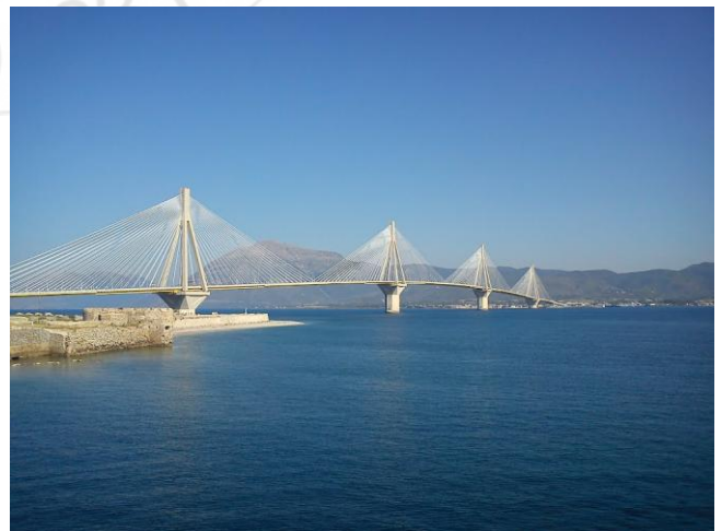
Figure 1: The largest cable stayed in Europe
