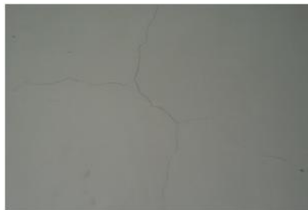
Figure 1: Plaster crack
