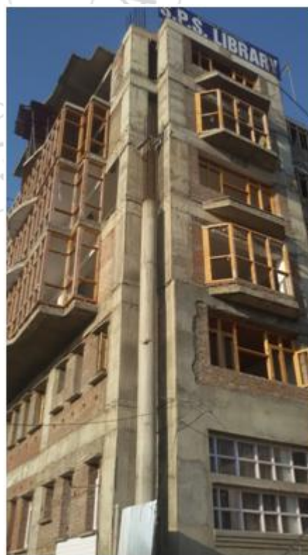
Figure 3: Slender columns at building corner
