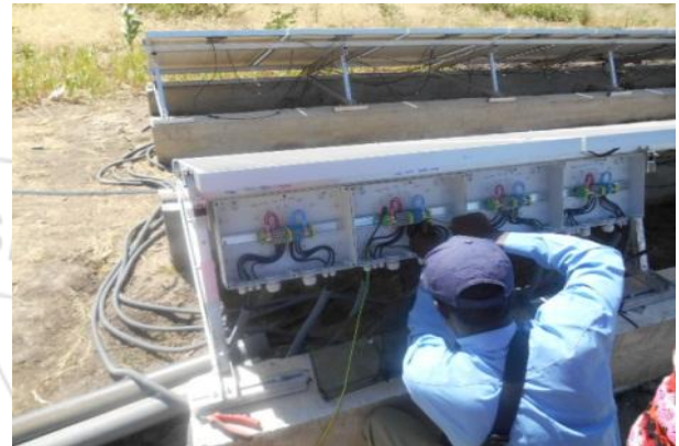
Figure 9b: Fixation of PV panel cables
