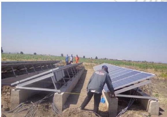
Figure 9a: Fixation of PV panel cables
