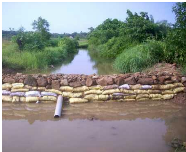
Photo No.3: construction of Vanrai bandhara
