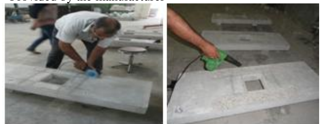
a: Removing the weak layer surface b: Cleaning the slab surface
