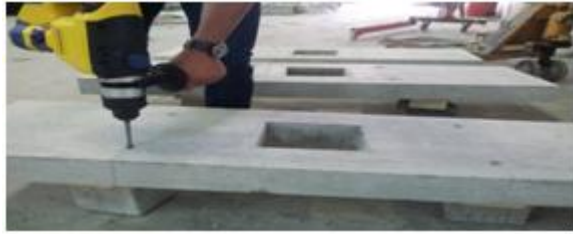
Figure 4: Making holes in RC slabs
