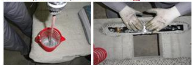
c: Mixing the epoxy materials d: Applying of CFRP strip
