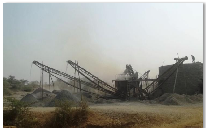
Figure 11: Working crusher at the mine site.
